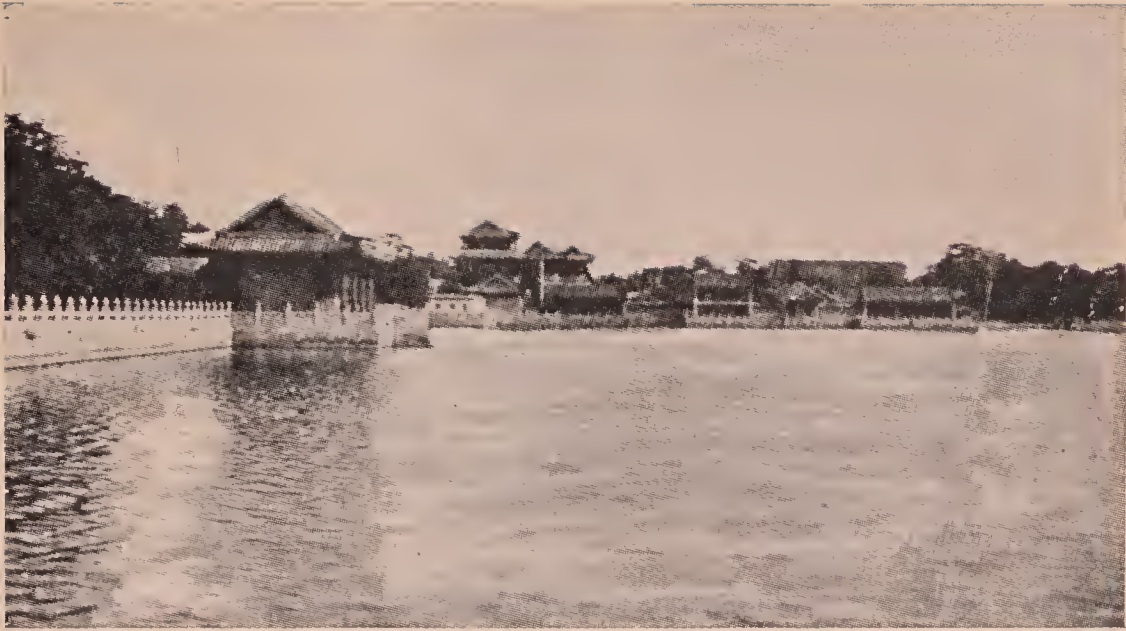
East Side of the Lake inside of the Summer Palace
